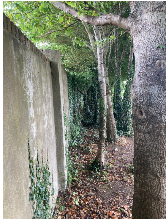
Image 4: Trees nearest the boundary wall are set back from the wall by 500mm on average.
