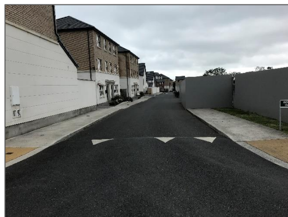
Figure 3.8 – Thornberry Road (Northern Boundary)
